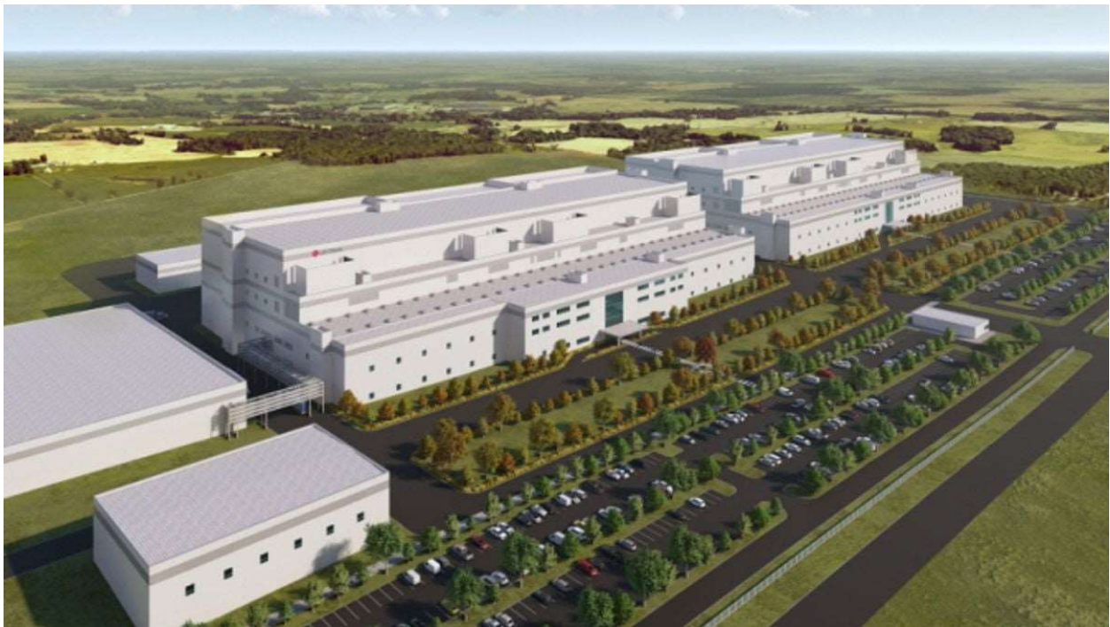
A model of LG Chem's planned production site in Clarksville, Tennessee. Courtesy of LG Chem
