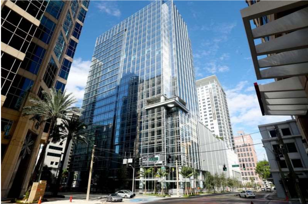
The intersection of Las Olas Boulevard and Southeast Third Avenue, site of the former Broward College downtown campus, as seen late last year. It is now home to The Main Las Olas, a mixed-use office, residential and retail building in the center of the city's financial and entertainment district. (Susan Stocker / South Florida Sun Sentinel)
