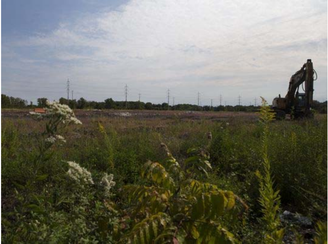
The former Evraz Claymot Steel site, a fallow 425-acre property, could offer Delaware's best chance of landing Amazon's second North American headquarters. (Photo: Jerry Habraken, The News Journal)
